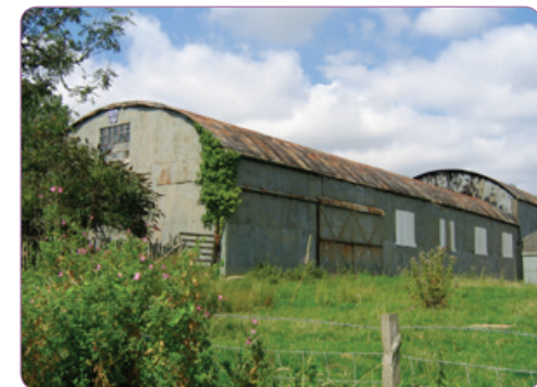
A typical mid 20th century shed, with a curved profile to the roof which resembles those used for iron-framed Dutch barns that date back to the late 19th century. (© English Heritage)
