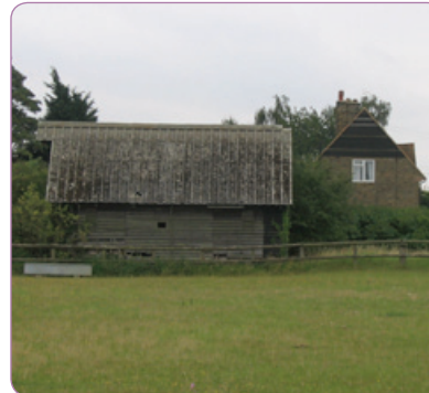
This is one of a group of rare surviving inter-war smallholdings at Thong close to Gravesend, now included within the conservation area of the village. (© Kent County Council)
